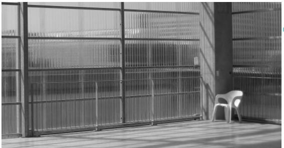
corrugated plastic panels
